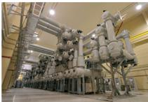
Figure 2: Typical GIS building and indoor switchgear.
