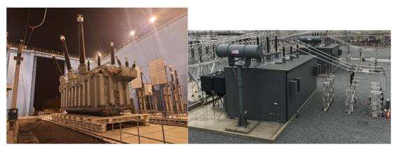
Figure 3: Typical transformers (righthand image with a noise enclosure)
