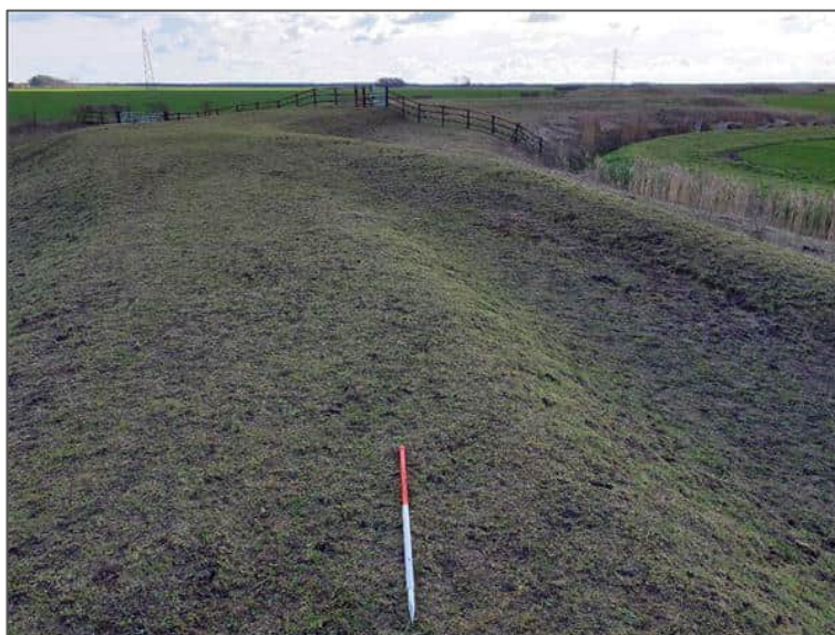
Plate 24: Section of sea wall recorded by LiDAR NGR 534065, 337047
