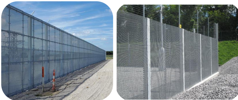
Figure 4.4: Typical examples of external fencing
